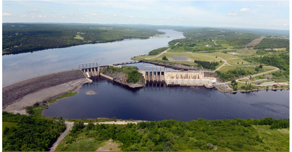
The Mactaquac Hydro-Electricity Generating Facility, 2014. Photo credit: NB Power.
